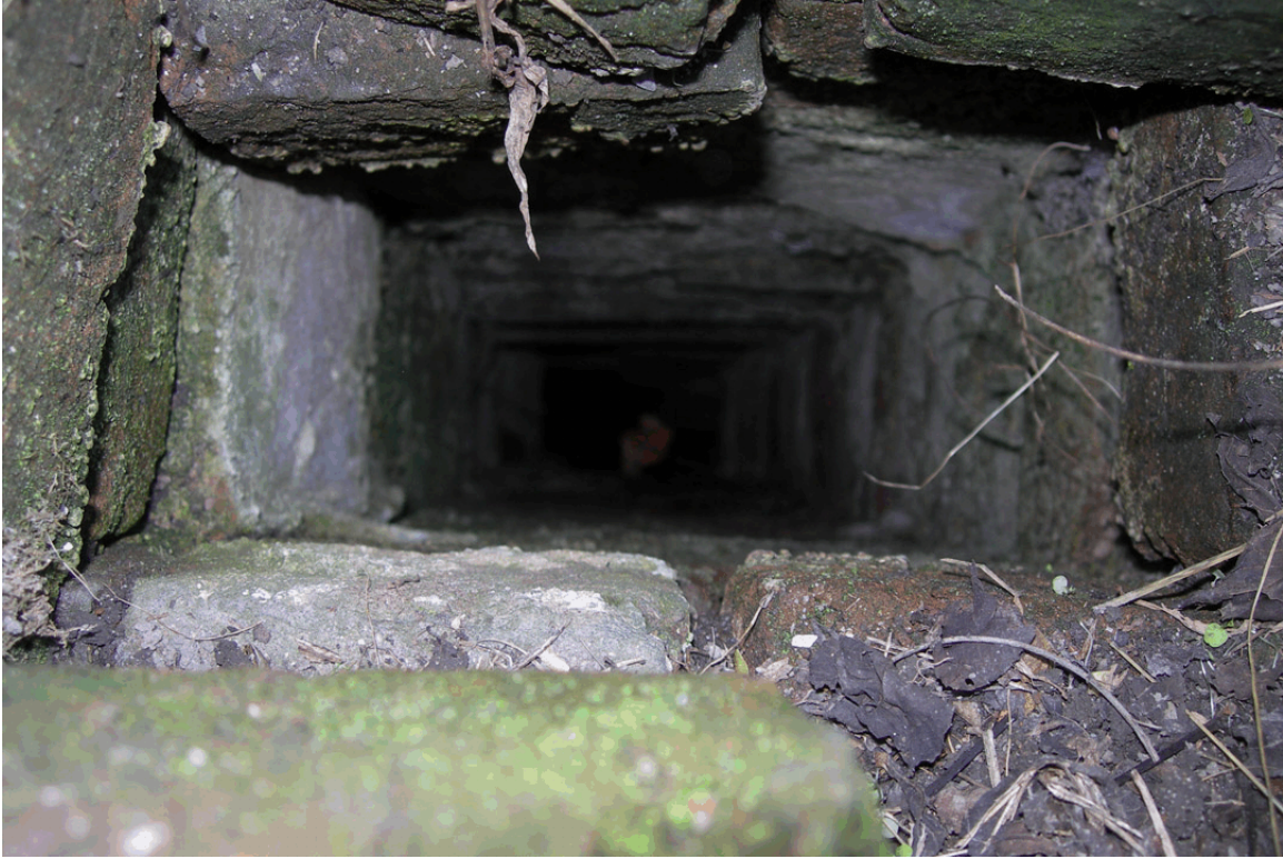
Figure 5.57. Detail of icehouse air vent.
