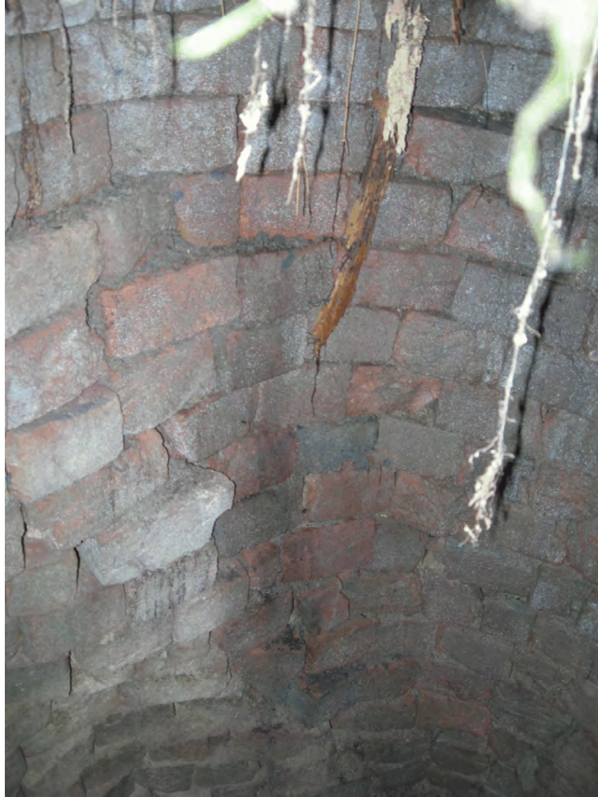
Figure 4.12. The well (note the inward bowing of the wall).
