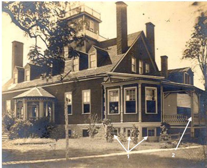
Figure 4. This view of the mansion was made during the Specht ownership period (1891-1906). The frame addition is on the right, against the east wall of the original mansion. 1. Basement windows in addition. 2. Post which may have been supported by the pier designated Feature F9-10. (Photo from the Gunston Hall Archives.)
